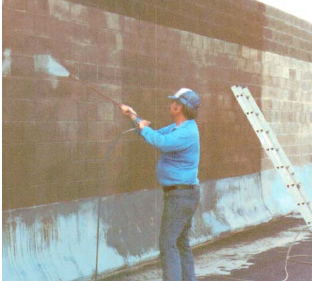
MA/CON BEING APPLIED TO A CAL-TRANS CONCRETE BLOCK SOUND BARRIER WALL
